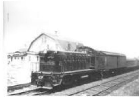
Mid-1940s: Southbound Lackawanna train switching milk cars at Dairymen's League plant north of Warren St. Jim Frey photo
